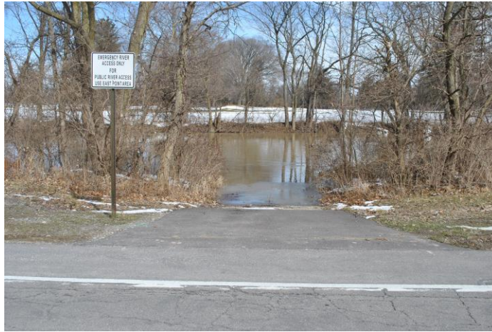
Emergency River Access (East Main Cross Street)
