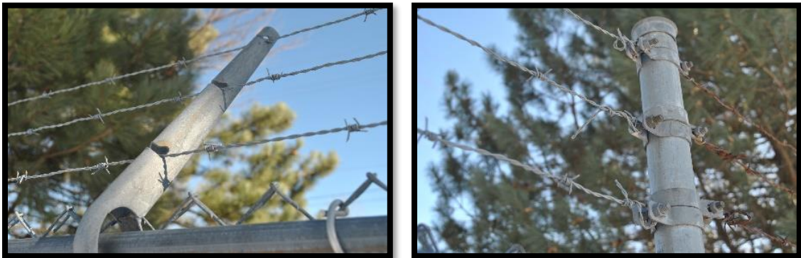
Fence Posts and Caps at Cooper Pond
