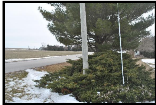
Cable covered with PVC pipes
