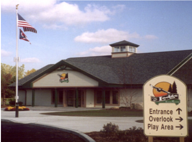
The Lodge at Riverbend is located in The Meadows area on TR 208
